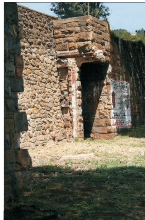
EVIDENCE OF VANDALISM, RECENTLY RECORDED IN THE ST JOHN ROAD ENCLAVE.
