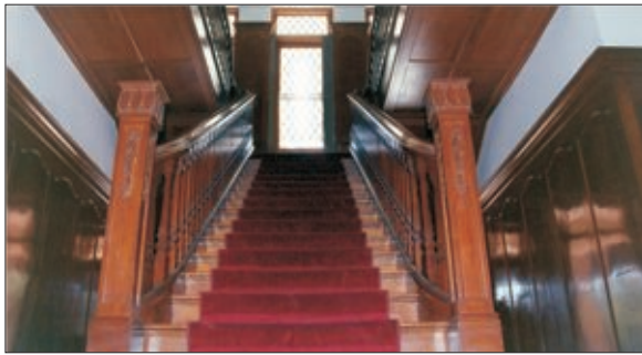
ORIGINAL NO RECORD (BELEIVED TO BE HOWDEN) BEFORE 1919, WILLIAM PAYNTER 1923 (VERANDAH ADDITION) 43 ST DAVID ROAD
