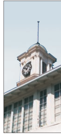
CLOCK TOWER CUPOLA
