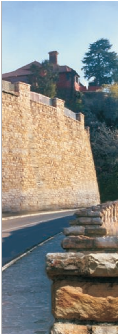
THE MUNRO DRIVE, NAMED AFTER JOHN MURO*, INITIALLY ERECTED 1919 IN SET DRY (STACKED) KOPJE STONE AND RECONSTRUCTED AFTER ITS COLLAPSE IN 1938, THIS TIME USING DRESSED KOPJE STONE SET IN MORTAR.
